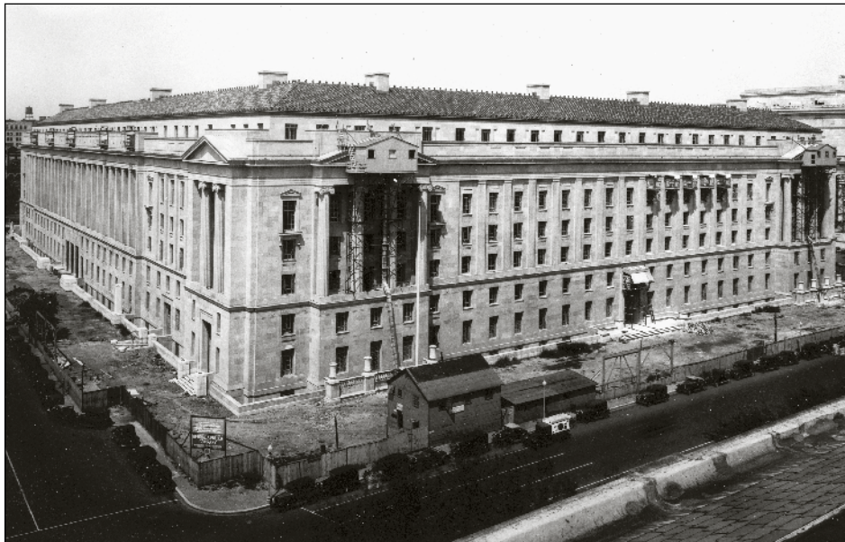
Construction photograph taken August 1934, showing the 10th Street and Constitution Avenue fronts of the building. Note the platform along the parapet on the 10th Street side and the pediments on the Constitution Avenue side for the carvers working on the sculptural decoration of those areas. Collection: National Archives, Audiovisual; photo no. 121-BCP-138B-15.
